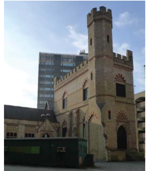
The Grade II listed Surrey Street Pumping Station is on the Heritage at Risk register
