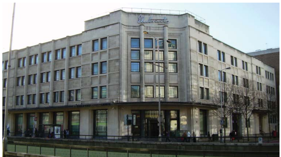
Electric House, Wellesley Road, Grade II
