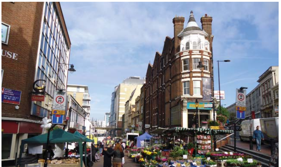
52-54 High Street (Millets building) at the sharp corner between Surrey Street and the High Street where there are significant land level changes
