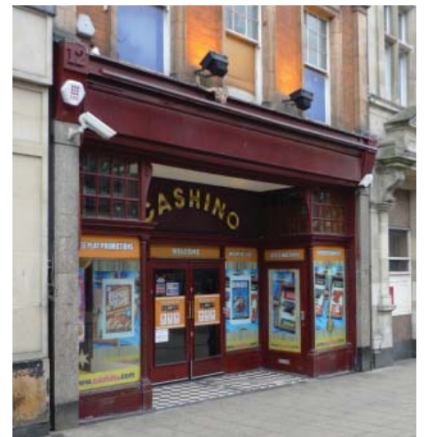
12 High Street: traditional style timber shop fronts
