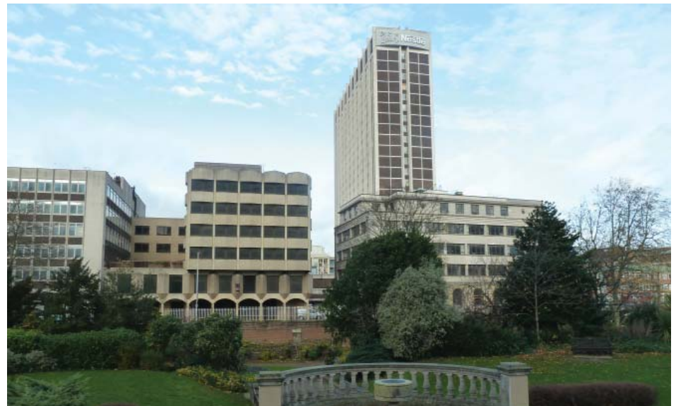
Segas House from the Queens Gardens, looking north
