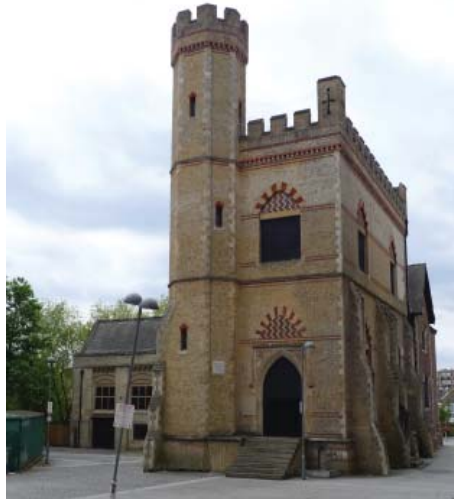
Surrey Street Pumping Station, Exchange Square, Grade II
