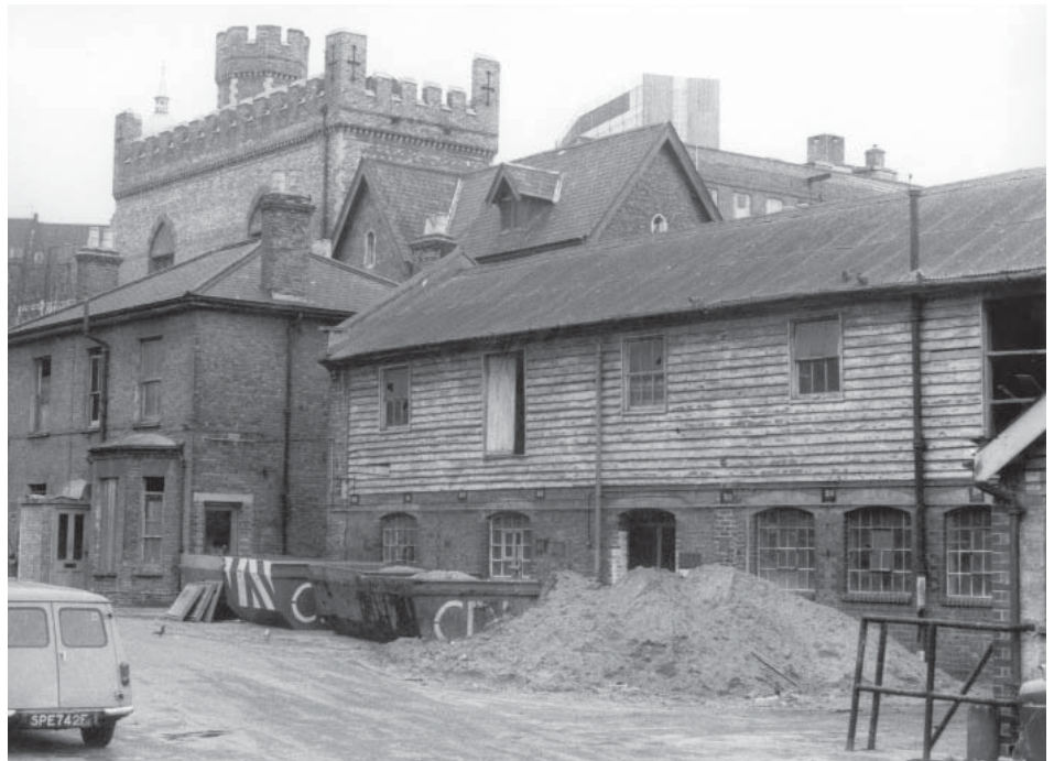
Historic photo c.1970s of the Surrey Street Pumping Station, the former railway station engine house, can be seen in the distance. The buildings in the foreground of this photograph have been demolished.
