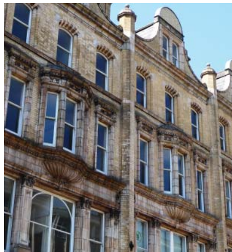
1890s commercial development, High Street
