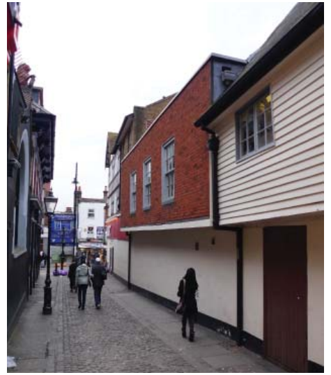
The rear of Numbers 11 and 13 Crown Hill, from Bell Hill
