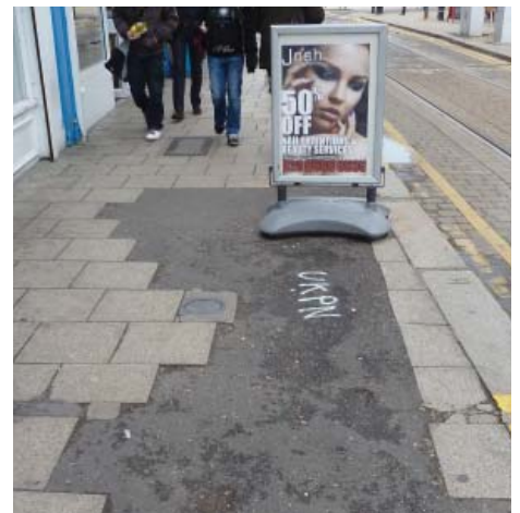
There are examples of poor maintenance of surfacing of footways and roads.
