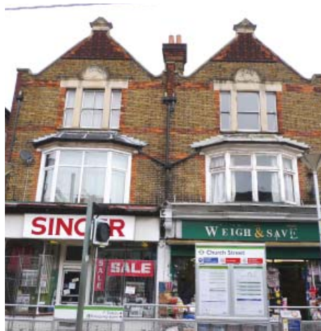
Late Victorian ornament and some surviving shopfront features, numbers 90, 92 Church Street
