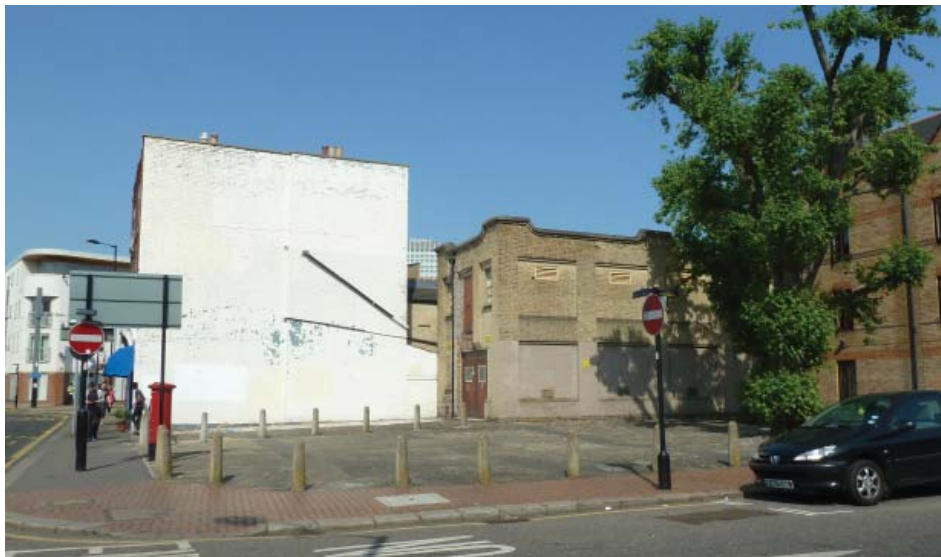
Open space in front of the substation at the corner of Church Road and Church Street
