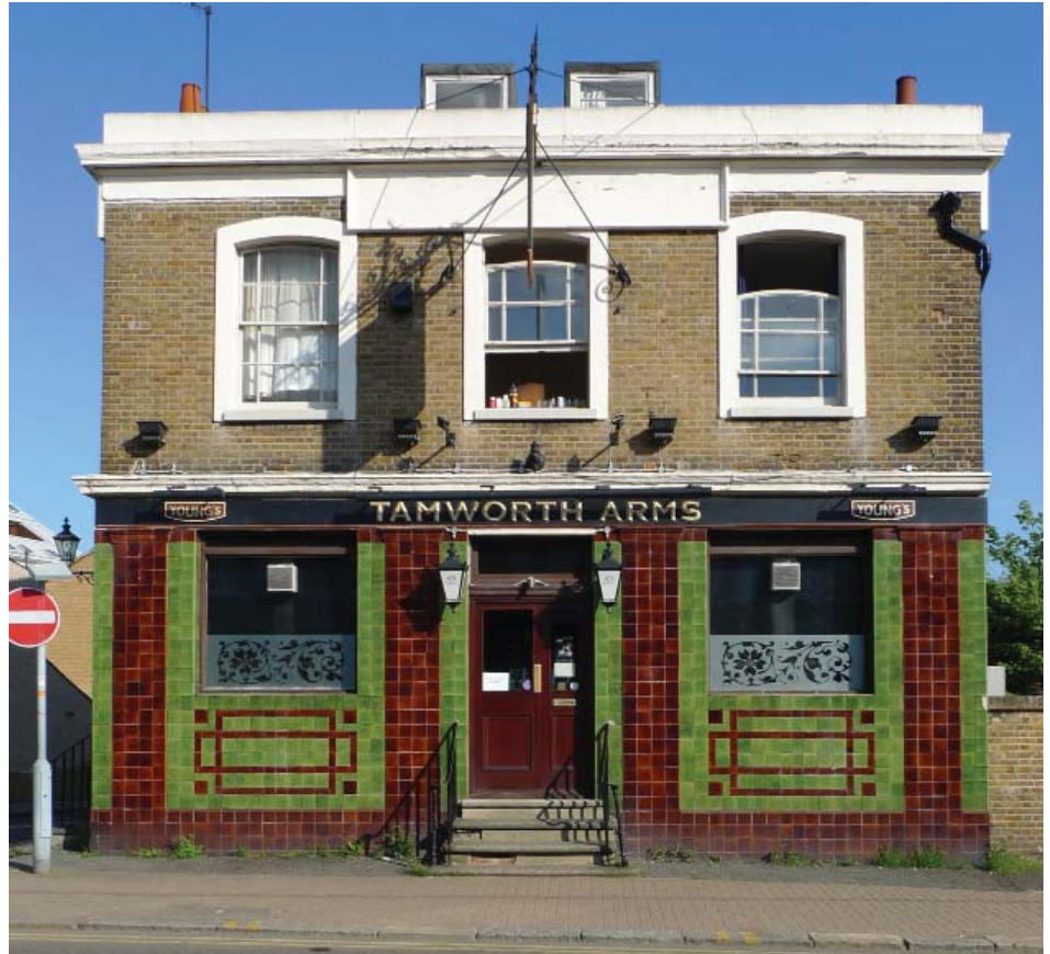
Locally listed Tamworth Arms public house
