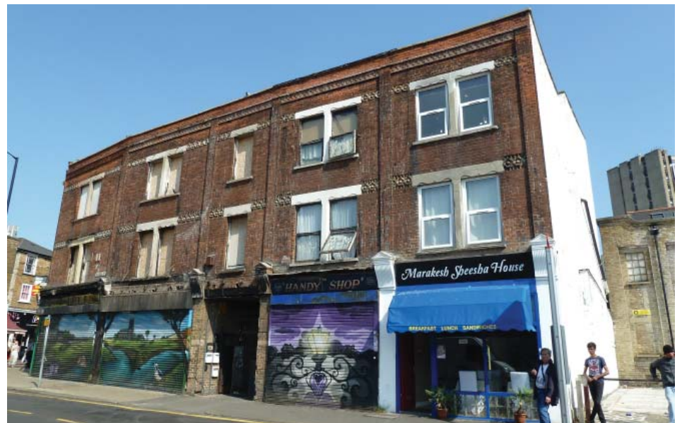
105-109b Church Street, facing Reeves Corner
