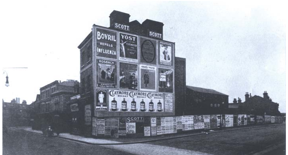
Corner of Church Street and Frith Road c.1900
