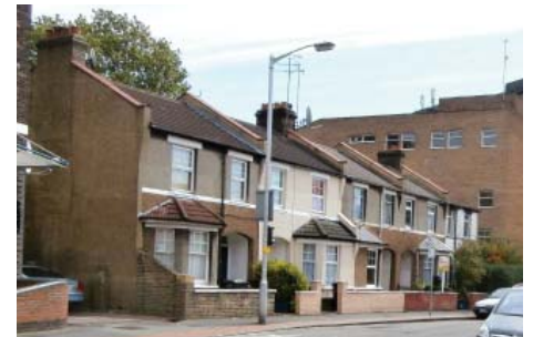
Rozel Terrace, a terrace of 1890s flats
