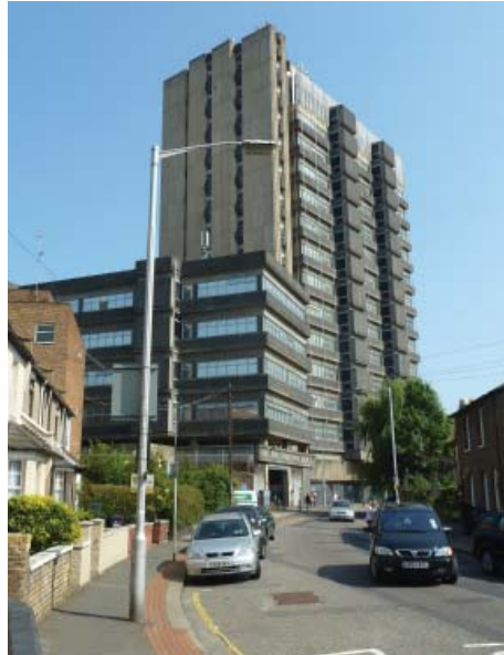
Ryland House has a significant impact on the setting of the conservation area
