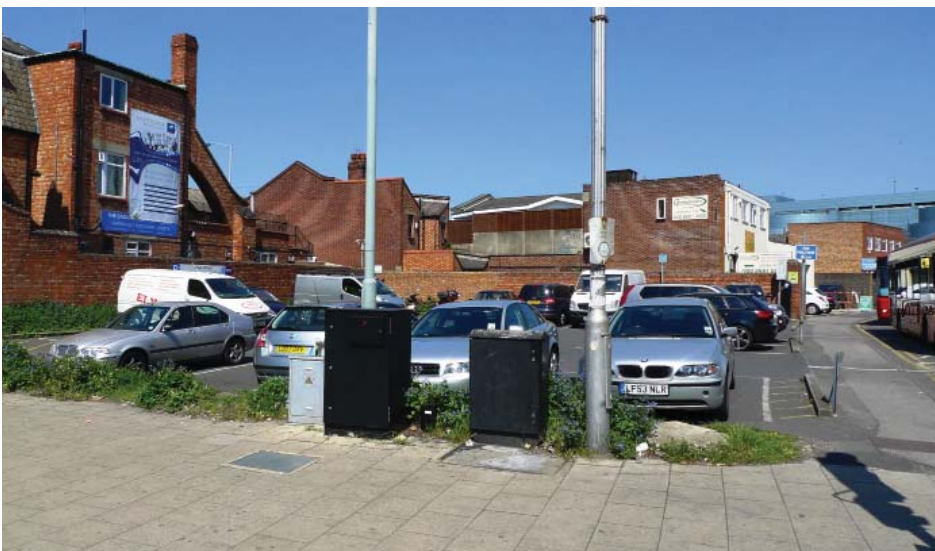
Car parks and yards off Drummond Road are poorly screened and harm the appearance of the conservation area. The lack of landscaping is an issue
