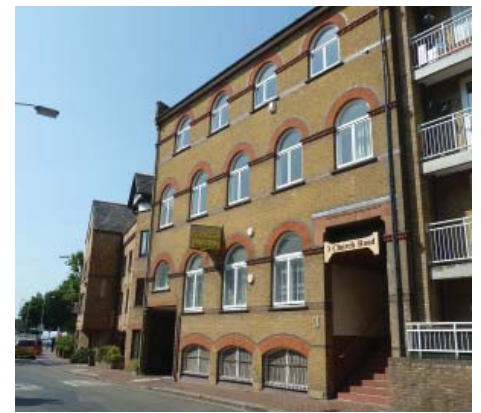
3 Church Road, a former Victorian shoe and boot factory
