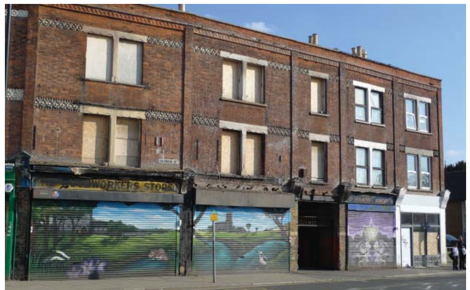
105-109a Church Street (locally listed), fire damaged and mostly vacant
