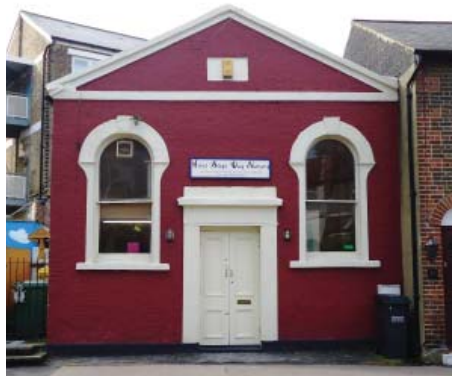
Former Wesleyan Chapel, locally listed, 26 Church Road
