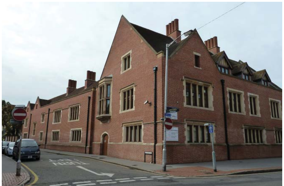
Old Palace Preparatory School building on the corner of Church Road and Old Palace Road. This high quality modern development was designed and built in 2001 by Porphyrios Architects. Built in red brick with crisp limestone dressings, it is of a contemporary design in a Tudor style. It respects and complements its important historic context and is a valuable addition to the Old Town area.
