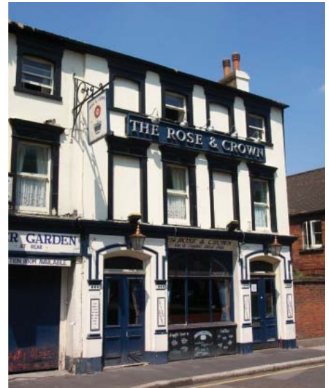
The former Rose & Crown public house
