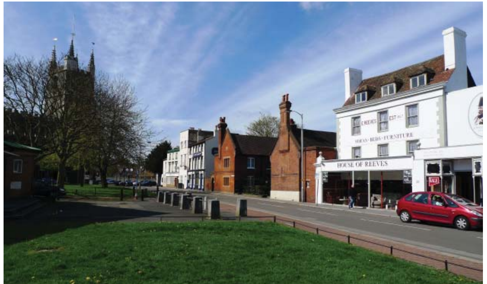
Buildings on the west side of Church Street form an important group with the Minster and create an interesting skyline
