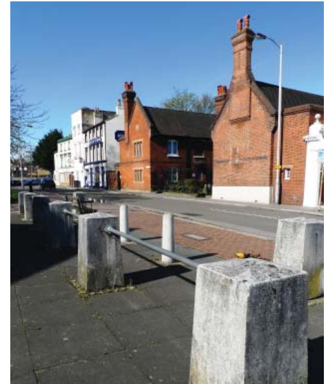
Oversized concrete bollards and rails outside the Church Hall which cause visual clutter in the street scene
