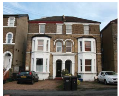
Pair of houses on Canning Road
