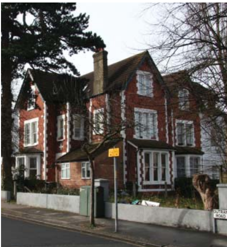
Number 180 Lower Addiscombe Road and number 99 Outram Road
