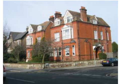
Numbers 179-183 Lower Addiscombe Road, within the Inglis Road LASC
