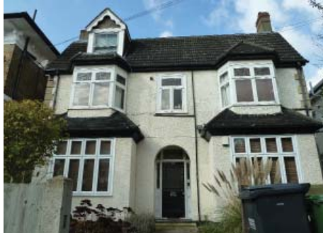
The original character of this building has been eroded by the introduction of render, the installation of uPVC windows at ground floor level and the installation of a dormer window to the front roofscape
