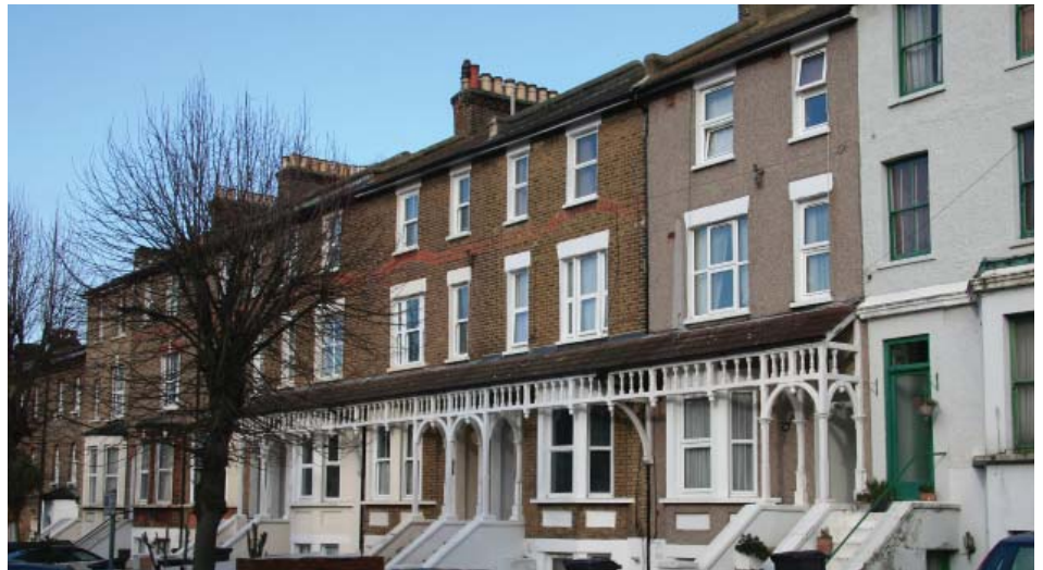
Terrace of houses at 76-82 Clyde Road with an elaborate timber porch
