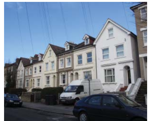
Consistent building lines on Clyde Road
