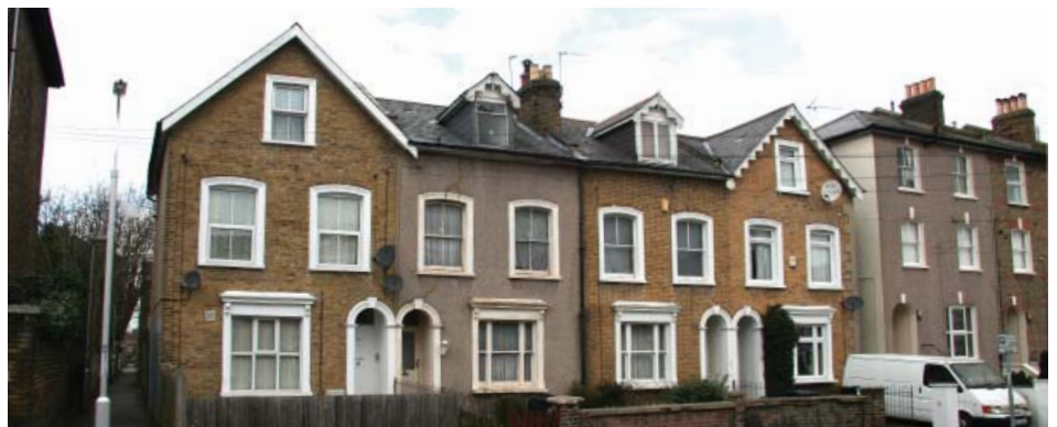
Short symmetrical terrace of four houses at 37-43 Elgin Road
