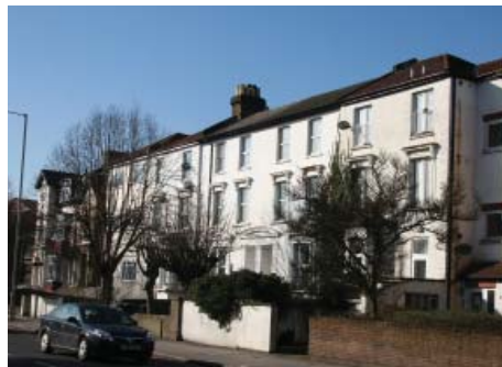
Consistent building lines on Addiscombe Road, set further back from the road than those within the East India Estate
