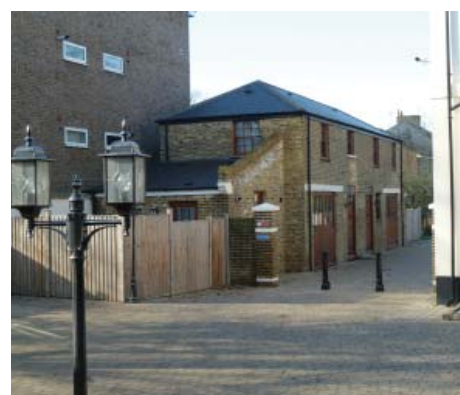
One of the historic Professor's Houses on Addiscombe Road was recently converted into flats, and the former Coach House was converted into two small houses. The work was carried out to a high quality and has resulted in an enhancement to the character and appearance of the conservation area.
