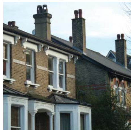
Houses on Clyde Road, typical of the architectural character of the East India Estate Conservation Area
