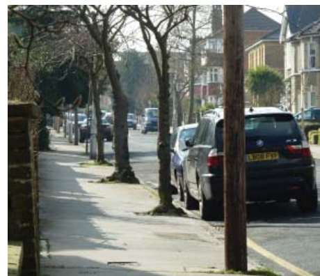
Asphalt surfaced footways on Outram Road
