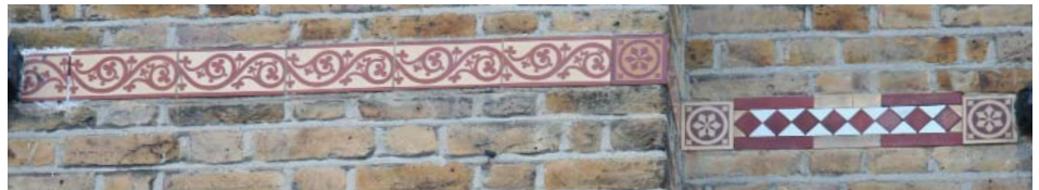
Architectural detailing of glazed tiles at 87 Elgin Road
