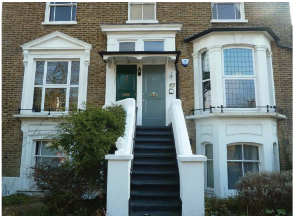
An examples where a property conversion has distorted the original symmetry of the building by creating an additional doorway
