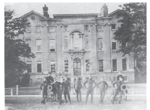
19th century photograph of Addiscombe House, when it was in use by the East India Company
