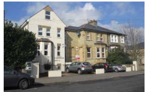
Oversized rendered extension (left) of a poor quality design and materials
