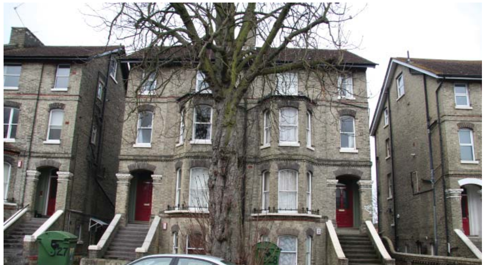
Street tree outside numbers 26-29 Canning Road
