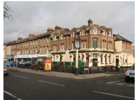
The Alma Tavern Public House and adjacent terrace
