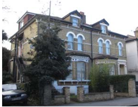
Two storey pair of houses on Clyde Road with central dormer windows
