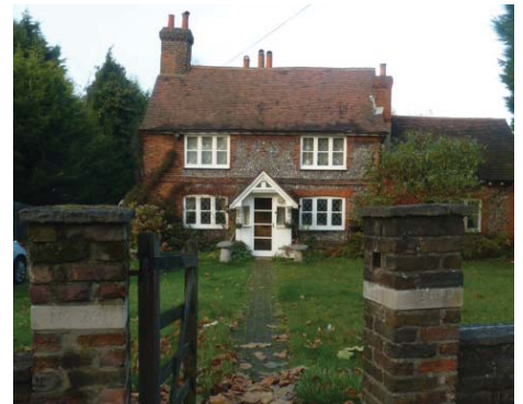
Grade II listed Addiscombe Farm, 281 Addiscombe Road
