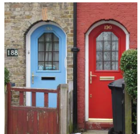
Part glazed timber doors - original design features
