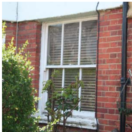
Rare surviving timber sash window
