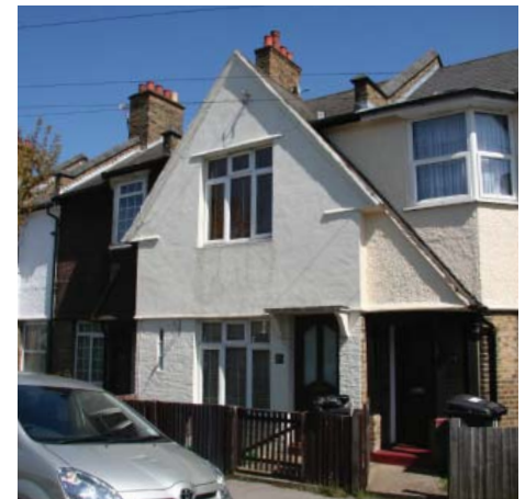
Recessed entrances located either side of a projecting gable
