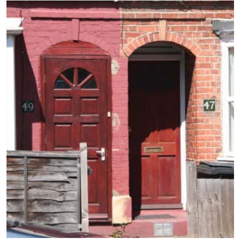
Infilled recessed porch and painted originally exposed brick
