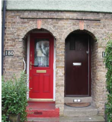
Well preserved recessed doorways and exposed brickwork
