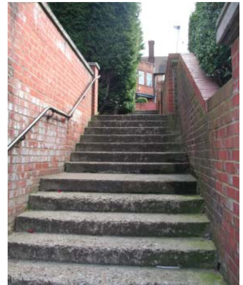
Isham Road public realm
