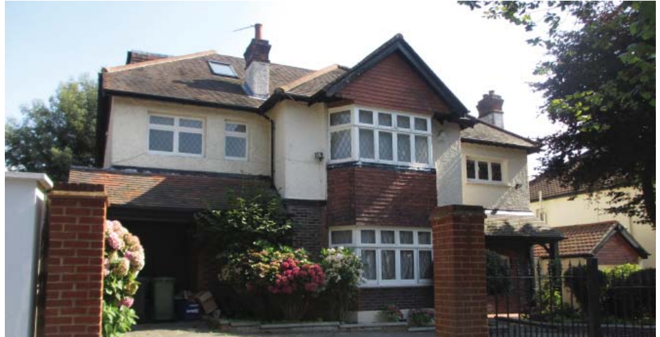
Two storey extension to 60 Ryecroft Road, set back from the front wall
