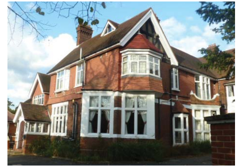
Gibson's Lodge Nursing Home - the building has been substantially extended to the south-west
