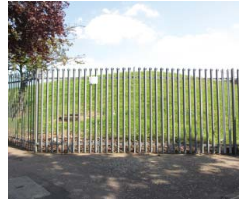
Unattractive palisade fencing marking the Norwood Reservoir boundary on Ryecroft Road
