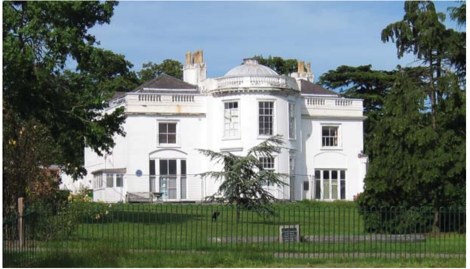
Front elevation of Norwood Grove Mansion
