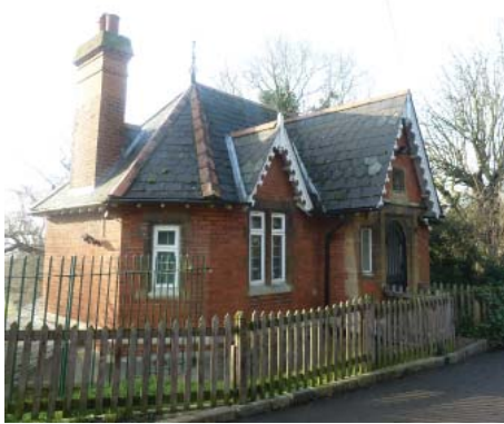
The Lodge viewed from Copgate Path
