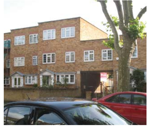
Modern development on Ryecroft Road, out of keeping with the established character of the area
