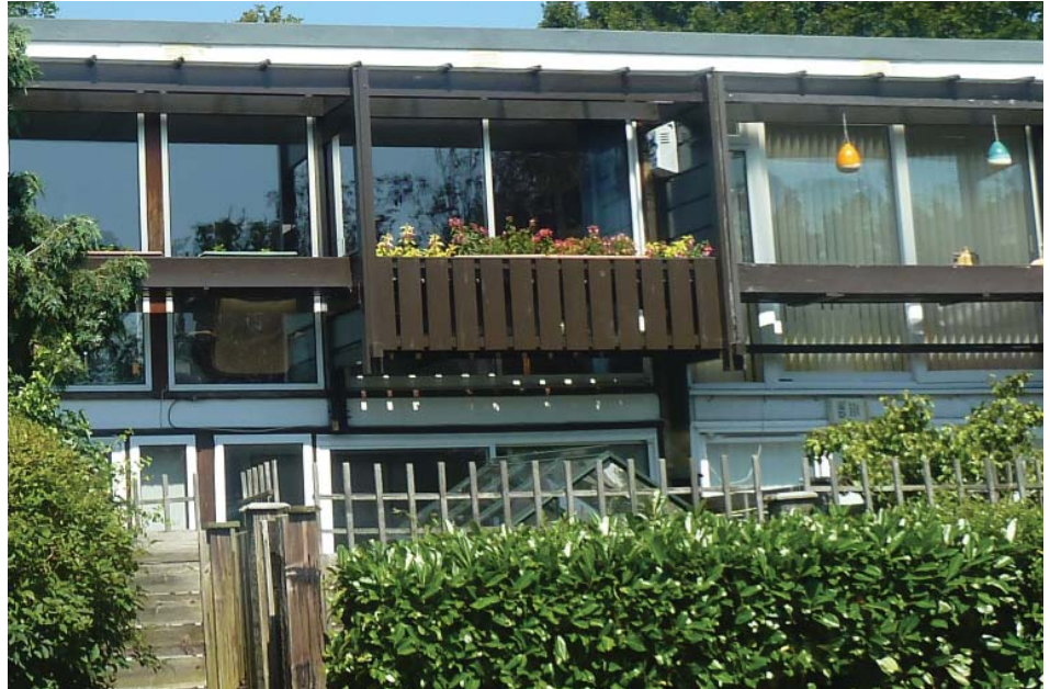
Timber balconies along a terrace at St Bernards
