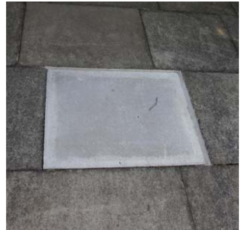
Examples of mismatching materials that have been replaced following works carried out by third parties
