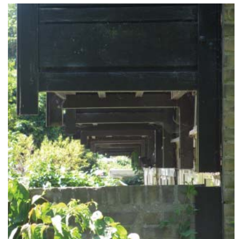
The underside of balconies
