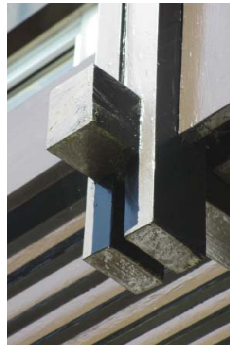
An example of the high quality construction detailing present
