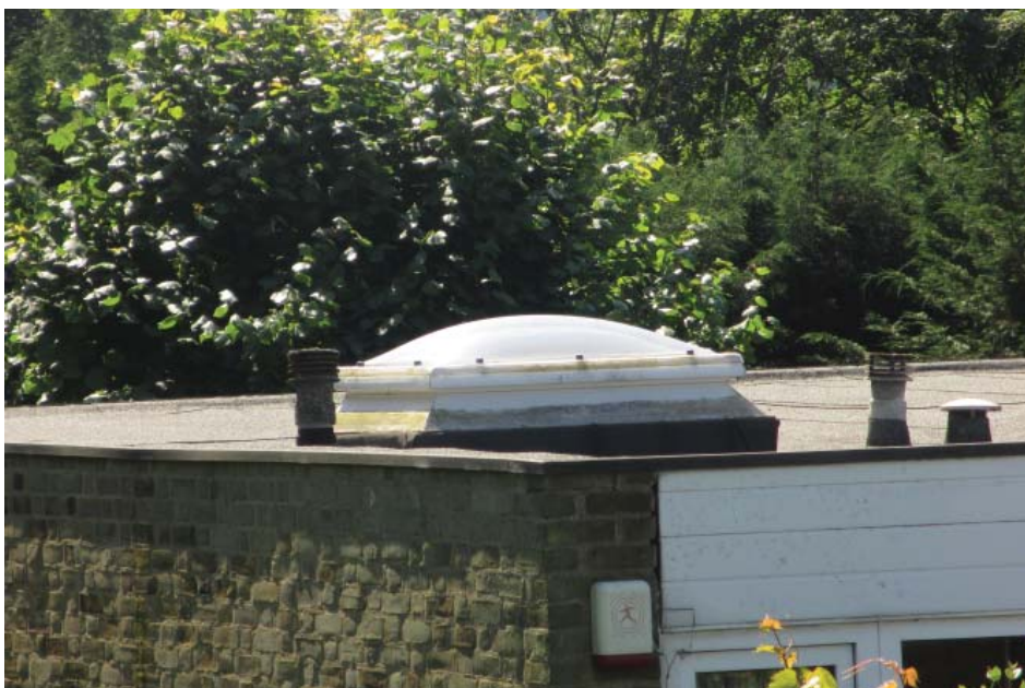
A replaced domed skylight that meets current Building Regulations
