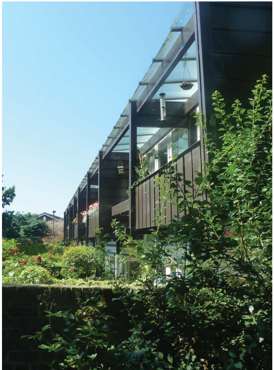
Well maintained southern elevation of a terrace of houses in St Bernards with important architectural features of balconies and timber panelling
