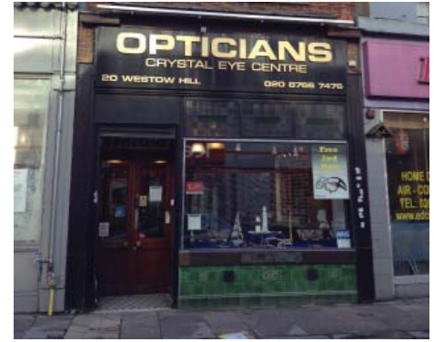
Historic shopfront at 20 Westow Hill
