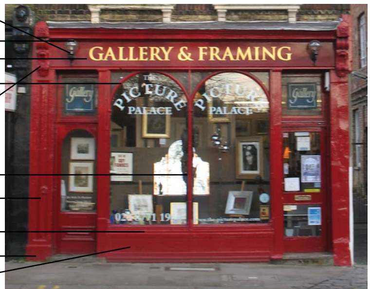
Surviving Victorian shopfront at 65 Westow Street, with labelled shopfront features
