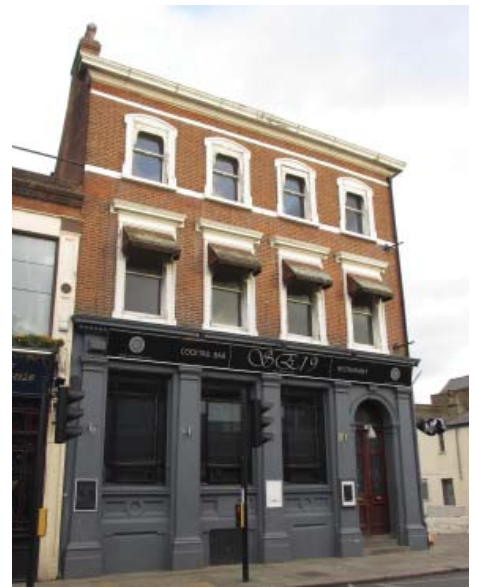
The Old Post Office, 35 Westow Street
