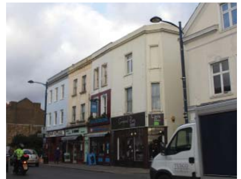
Three storey terraced buildings on Westow Street
