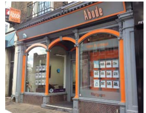
Historic shopfront at 80 Westow Hill
