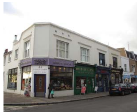
40-44 Westow Street, historic two storey early 19th century buildings
