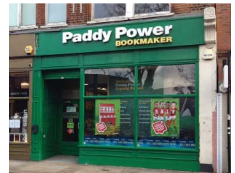
Traditionally designed modern shopfront at 47-49 Westow Street
