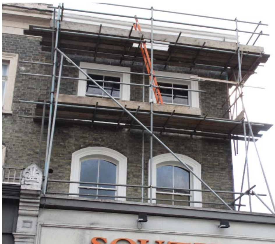
Historic features in the process of being repaired at 26 Westow Hill
