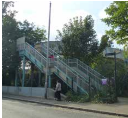
The existing bridge into Wandle Park
