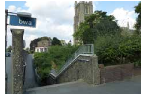
The existing subway does not create a pedestrian friendly public realm along Roman Way
