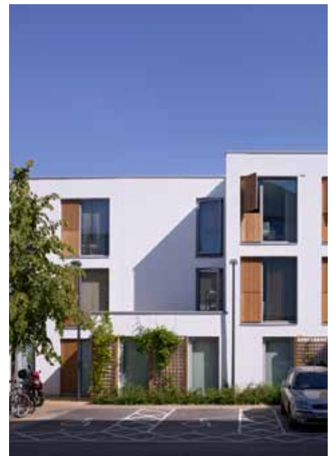
Car parking, bike parking and planting within developments, Arsenal, London - Allies and Morrison
