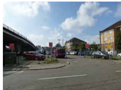
The existing Wandle Road car park
