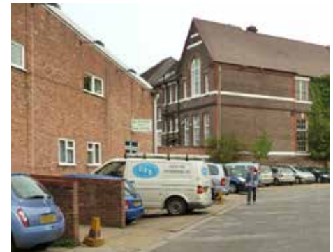
Existing site with locally listed former school in background
