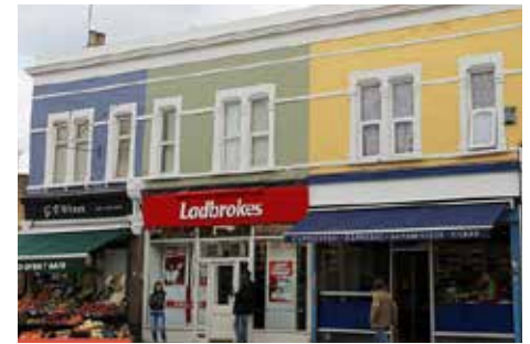
Before (top) and After (bottom) Leyton Shop fronts improvements and public realm scheme (Daily Mail)
