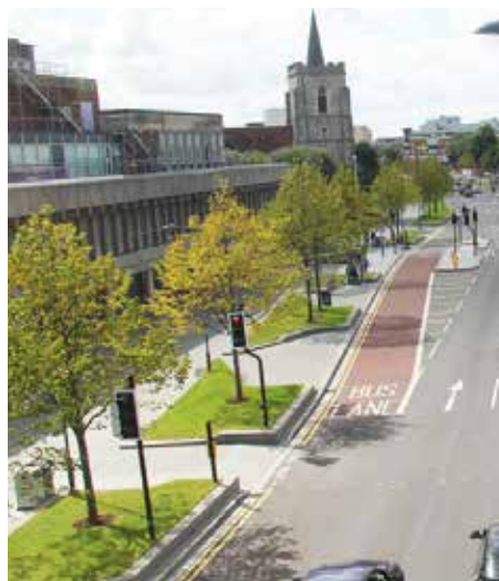
Heart of Slough project, creating a pedestrian friendly public realm at the side of a busy route (Spacehub)
