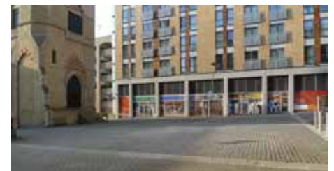
Existing public realm at Exchange Square with the Pumping Station to the left (see OT5 for more information). The green box is the non-operational Thames Water switching house. The retail units are unoccupied
