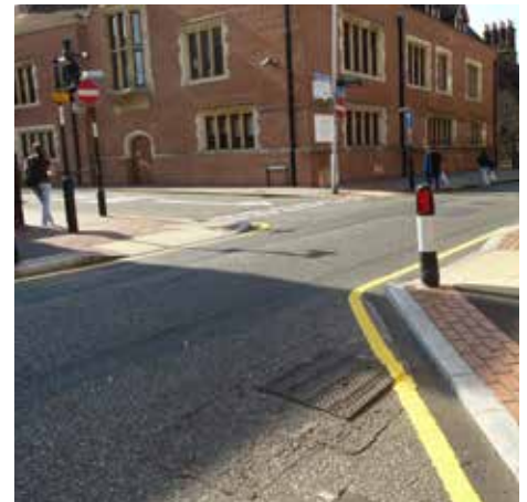
Existing crossing point at Old Palace Road, across Church Road
