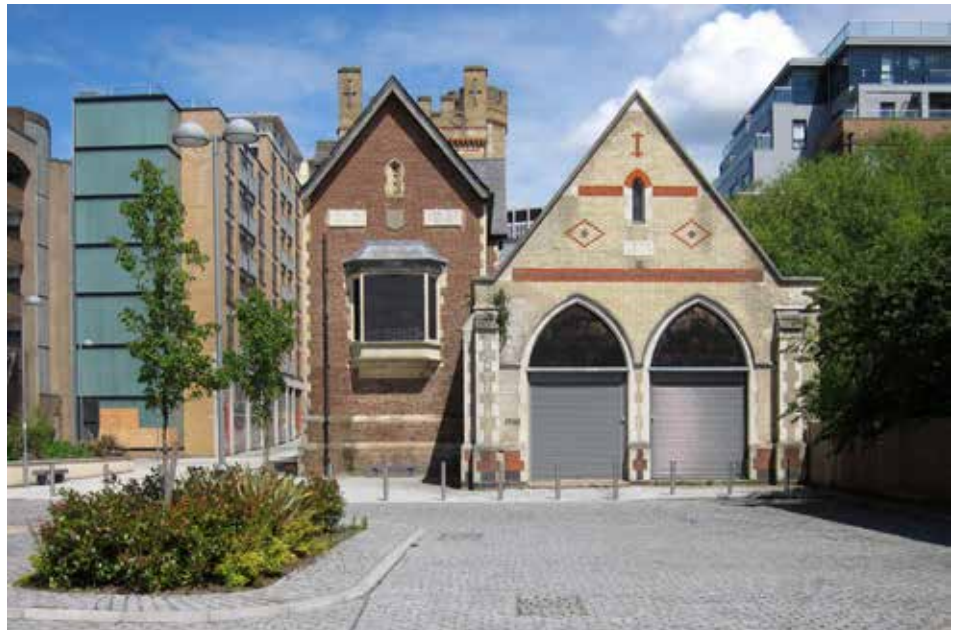
The rear of Surrey Street Pumping Station, from Charles Street
