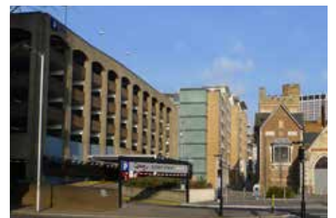
Existing car park and vehicular entrance
