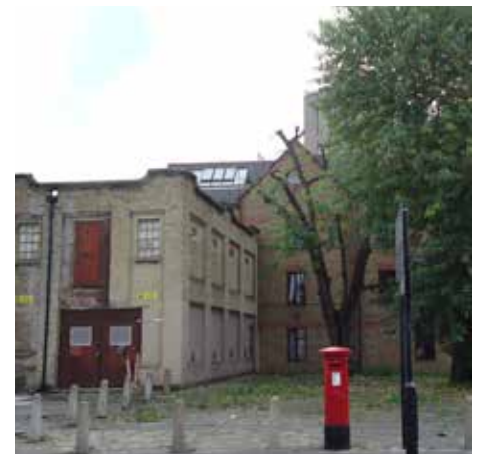
Existing public realm on Church Street and the electricity substation
