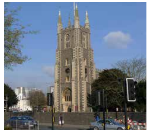
Roman Way and the subway compromise the setting of the Minster
