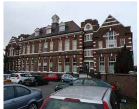
The former school has a car park in front, on Tamworth Road
