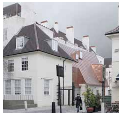
New Horizon Youth Centre, Somers Town, North London with copper extension (Adam Khan Architects)
