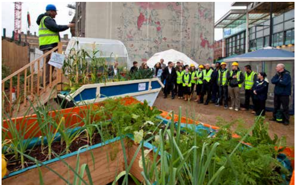
Temporary skip gardens during construction at Kings Cross. This project is ongoing and now has a pop-up cafe
