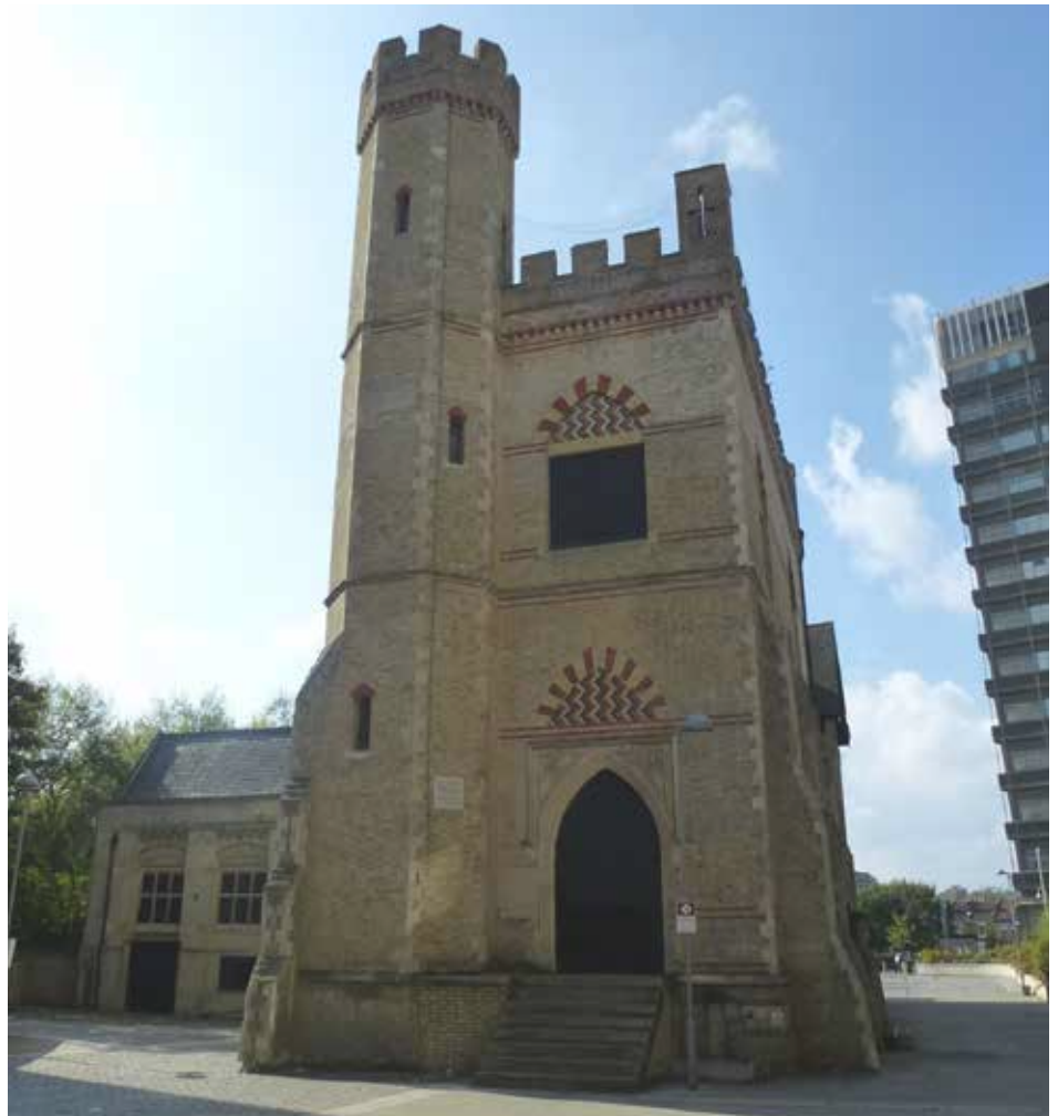
Surrey Street Pumping Station, Exchange Square
