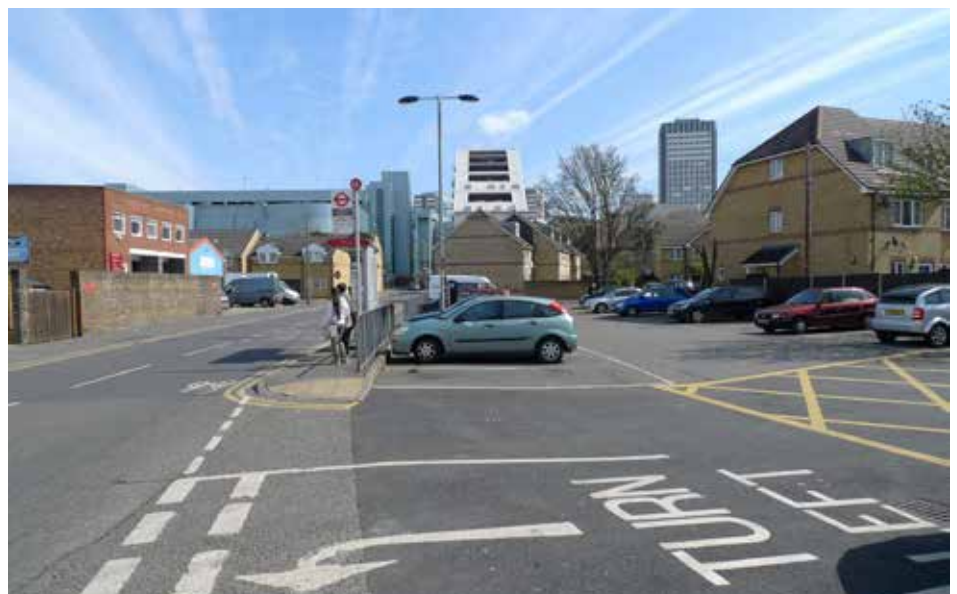
Drummond Road Car Park to the right, inactive frontage to the right on Drummond Road and the Central Centrale in the distance
