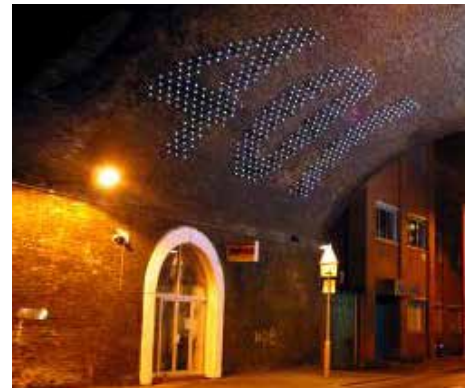
Creative lighting helps to make an underpass more inviting for pedestrians, Southwark Street
