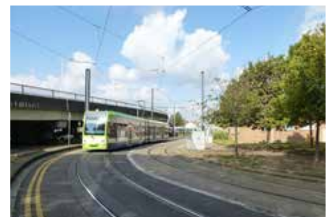
Existing tramways and the jubilee flyover
