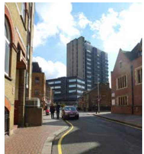
Church Road is the location of some of Old Town's office stock, Church House Business Centre (left side) and Ryland House in the distance
