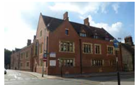
Infill development at Old Palace School in Old Town with scale and materiality that responds to the existing historic condition
