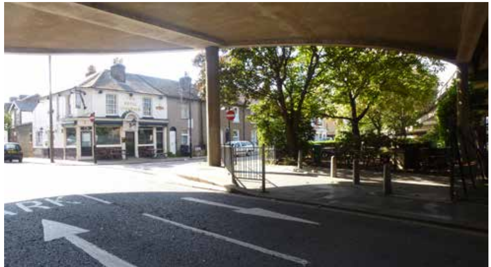
Existing Croydon Flyover undercroft with the beer garden of the Royal Standard
