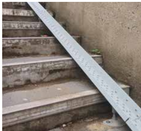
Wheeling channels, Old Barn Lane, Croydon
