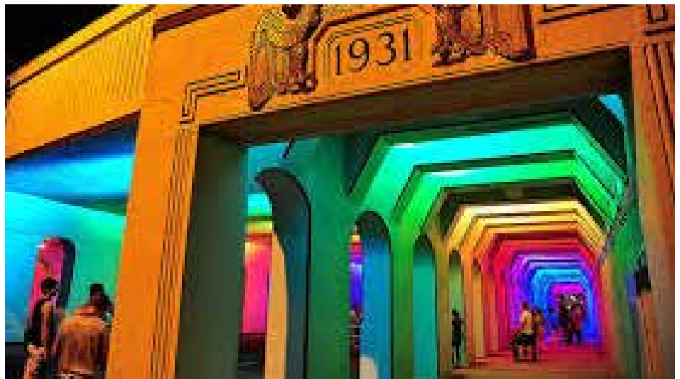
Creative lighting to improve a sense of safety at an underpass in Birmingham, Alabama
