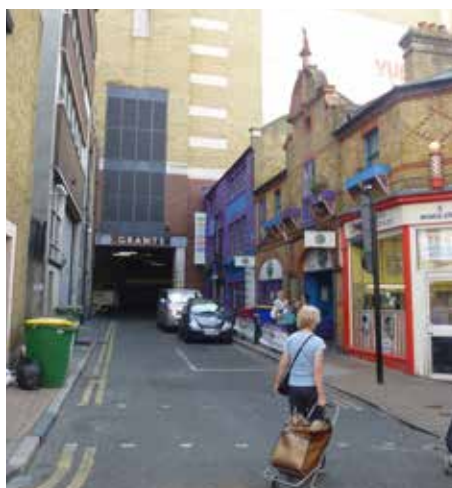
The service yard on Middle Street has a detrimental impact on the public realm
