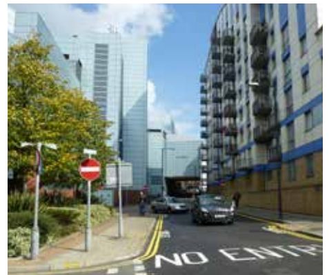
Existing route under the Centrale shopping centre
