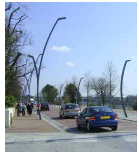
Shared surface treatment of the town's southern ring road. Space has been given back to pedestrians and used to plant street trees, Ashford.
