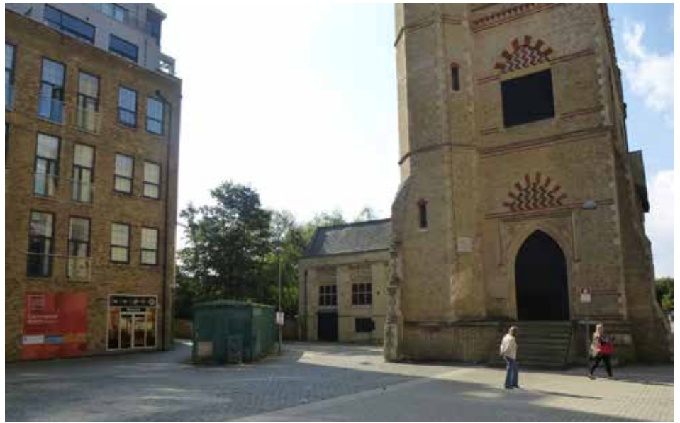
Surrey Street Pumping Station in Exchange Square
