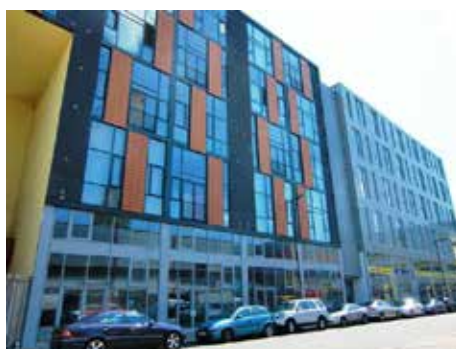
Issigonis and Morris House, Acton - live/work units which provide activity to the street
