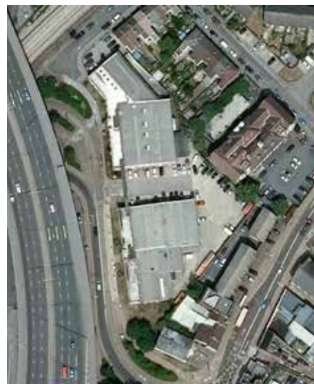
The existing Cairo New Road site (image 2013 Bluesky)
