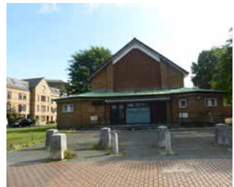
The existing public realm in front of the church hall is poor quality
