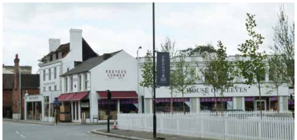
The temporary area of landscaping in place at Reeves Corner
