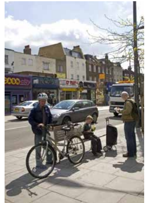
High quality street furniture and tree planting in the widened footways, Walworth Road (CABE). Elements of this scheme are useful precedents for Church Street
