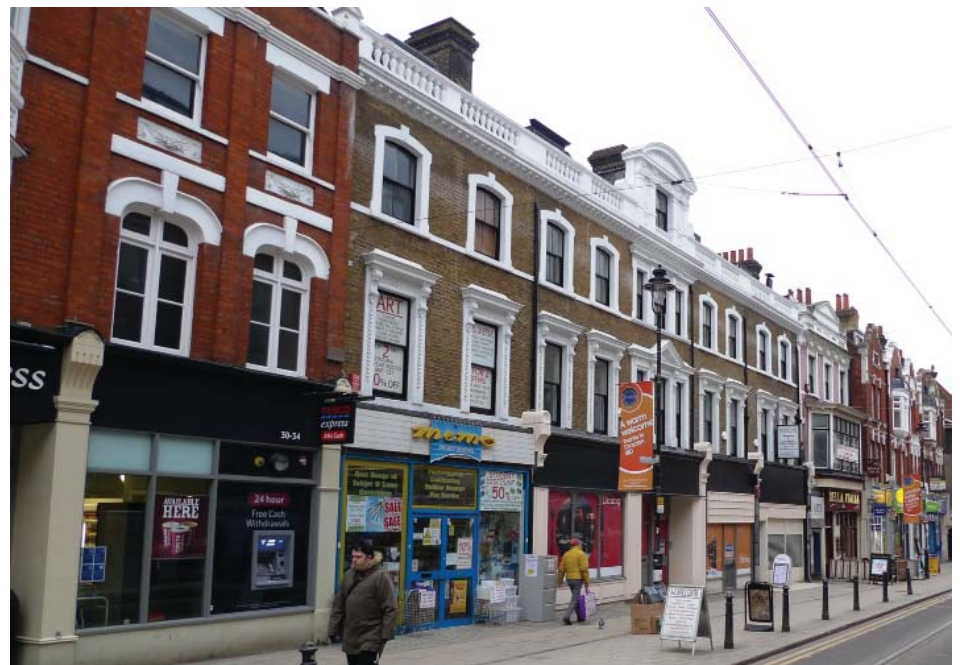
Terraced buildings on the north side of George Street
