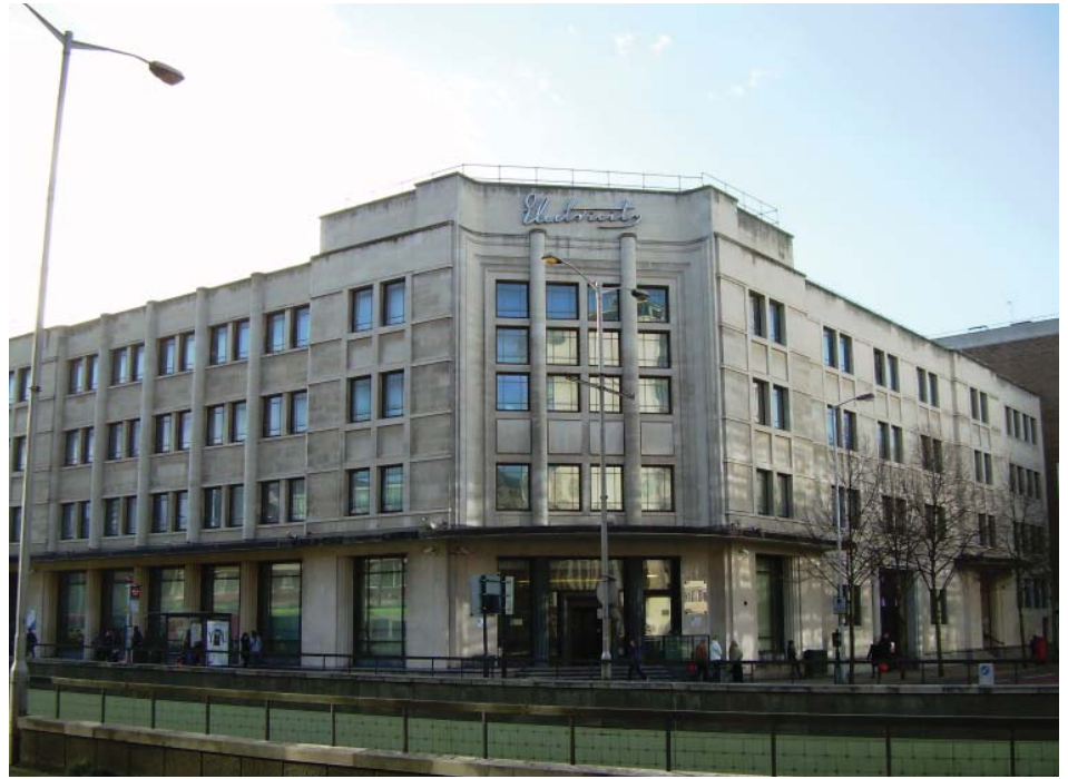
Electric House, Wellesley Road, Grade II
