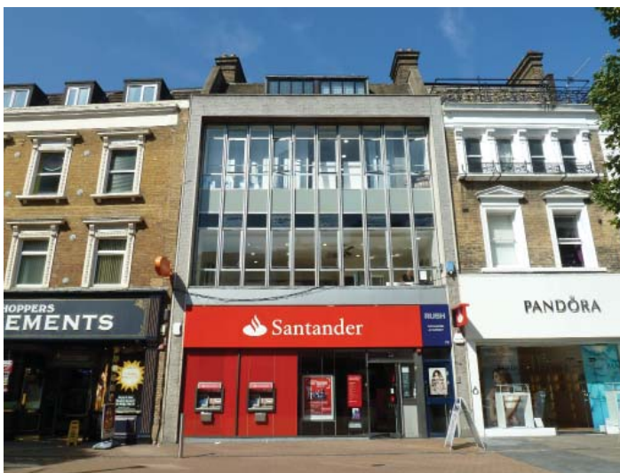
73 North End, a building that makes a neutral contribution to the conservation area's special character
