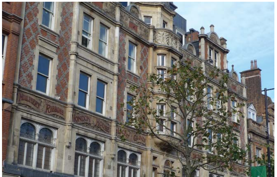
Historic facade to the former Grants department store, with delicate detailing and brickwork patterning (1894), Grade II listed
