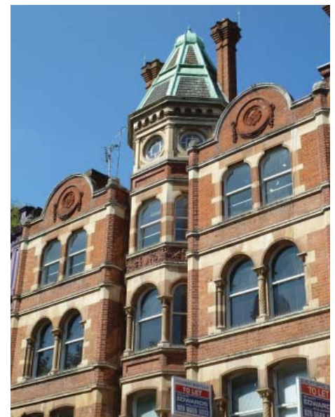
Detail of 32-34 High Street
