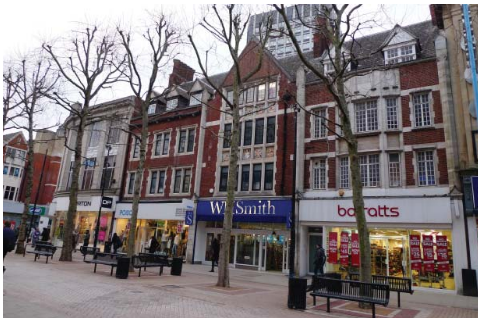
Tudor-Revival buildings on North End (numbers 32, 34 and 34a) with trees and public seating
