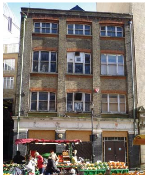
46 Surrey Street, the former Croydon Advertiser building, is currently in a poor condition
