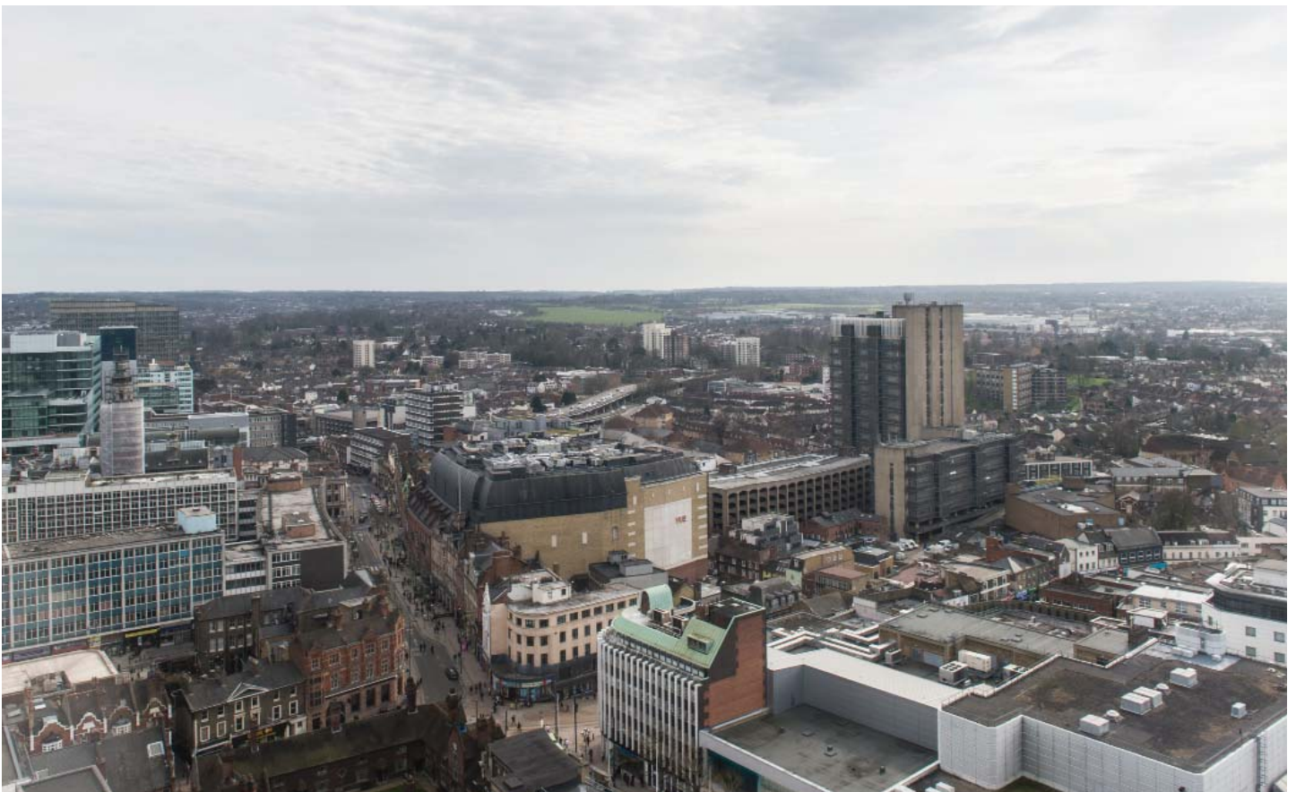
View of the central Croydon area from Centre Tower above the Whitgift Centre, looking south-west. The bulky massing of the Grants complex is particularly prominent as is Ryland House
