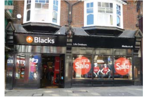
3-5 High Street: traditional style timber shopfront
