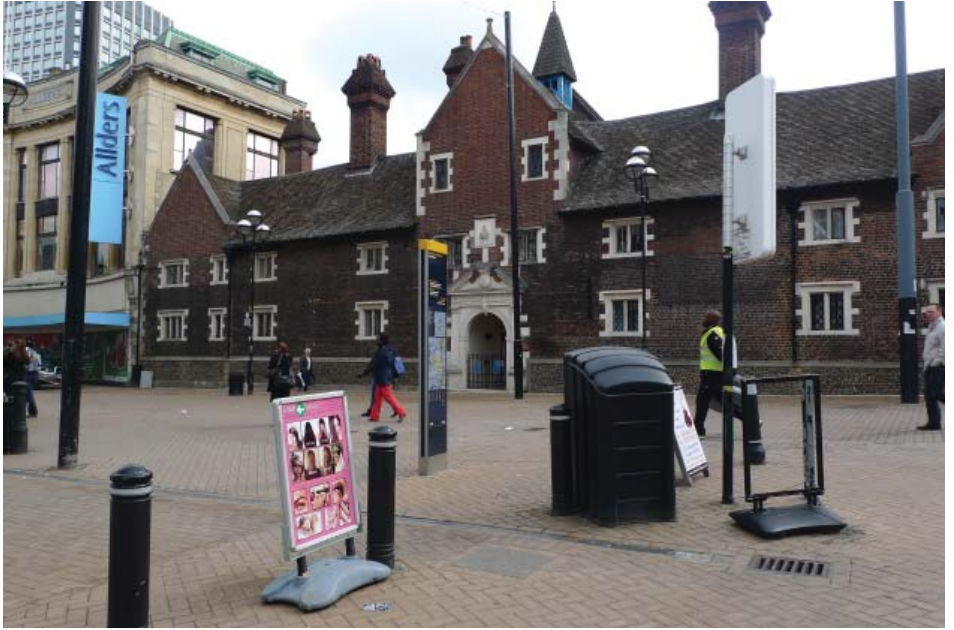
Some street furniture is intrusively sited and causes clutter to the streetscape
