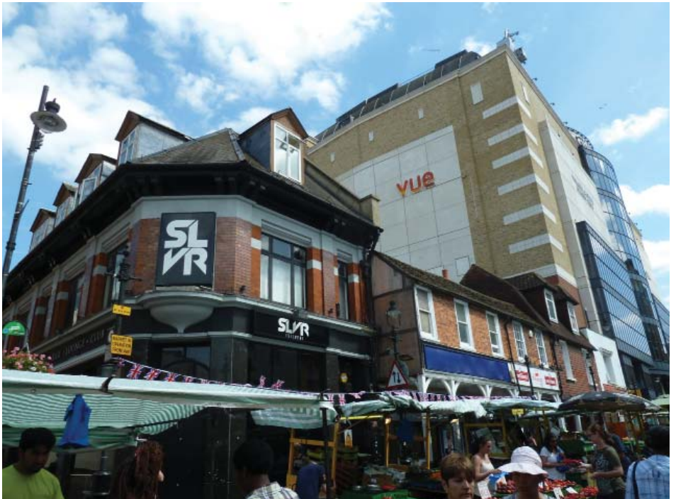
The rear of the Grants Complex has a harmful impact on the character of Surrey Street due to its overbearing scale
