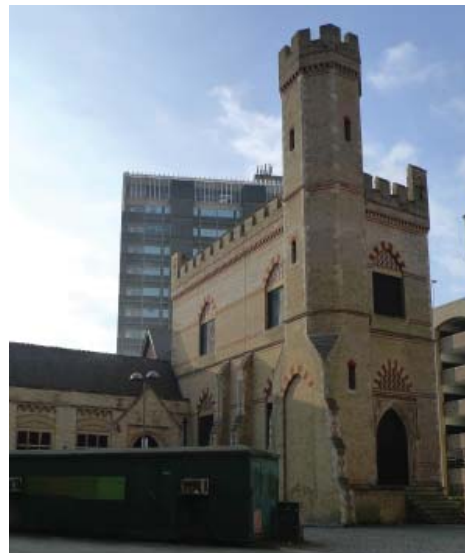
The Grade II listed Surrey Street Pumping Station is on the Heritage at Risk register
