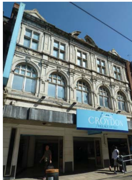
White terracotta facade, 5 George Street, former Allders department store
