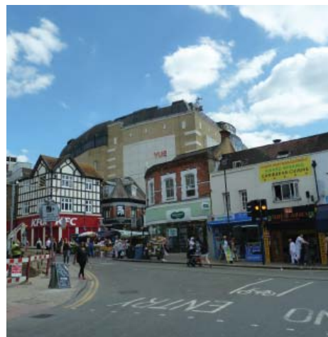
The eastern end of Church Street and the entrance to Surrey Street, showing the visual dominance of the rear of the Grants complex
