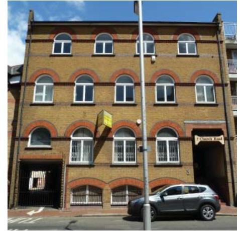
3 Church Road, a former Victorian shoe and boot factory
