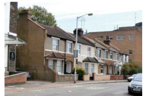
Rozel Terrace, a terrace of 1890s flats
