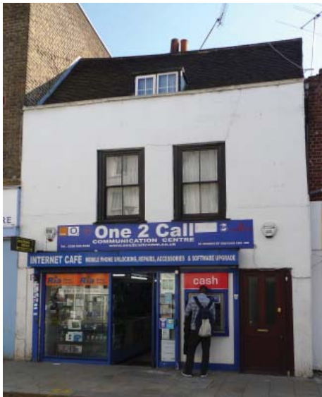
Grade II listed 91-93 Church Street
