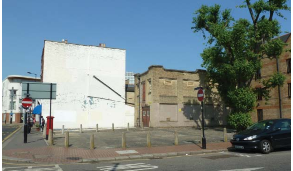
Open space in front of the substation at the corner of Church Road and Church Street
