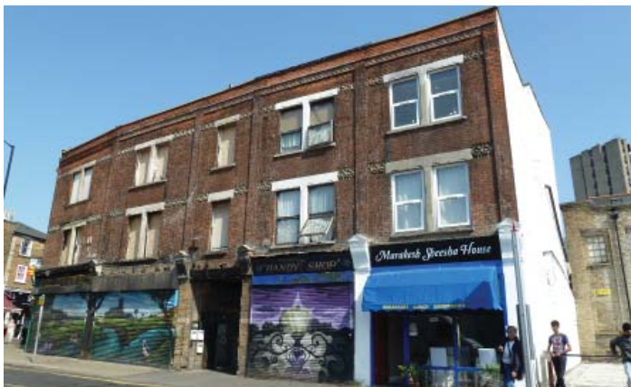
105-109b Church Street, facing Reeves Corner, which suffered fire damage during the 2011 Civil Disturbances
