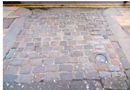
Crossover at 43-45 Church Street with granite setts and kerbs
