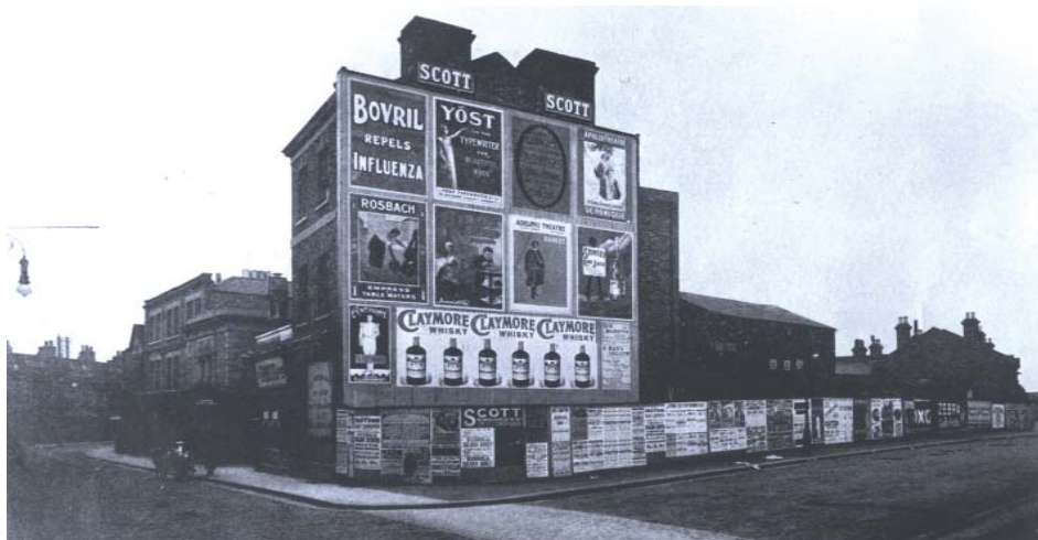
Corner of Church Street and Frith Road c.1900
