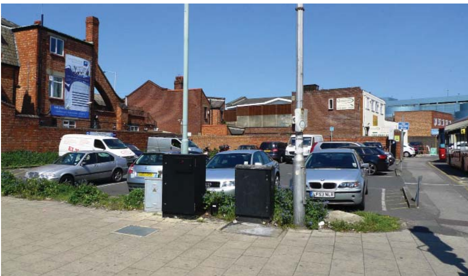
St Ann's car park on the corner of Church Street and Drummond Road is poorly screened and detracts from the appearance of the conservation area, there is also temporary signage located on buildings that further detracts from the appearance of the area
