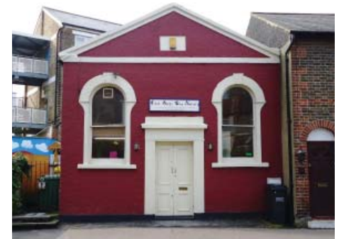
Former Wesleyan Chapel, locally listed, 26 Church Road
