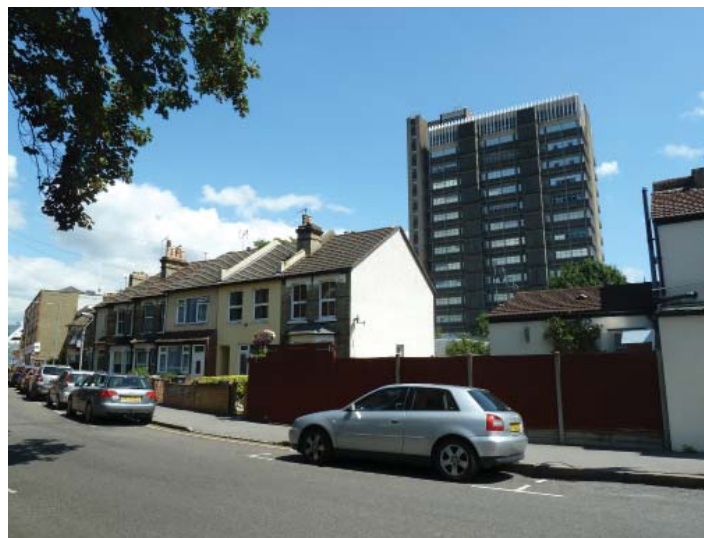
View of Old Palace Road, showing the dominant and negative impact that this 15 storey building has on the character and appearance of the conservation area
