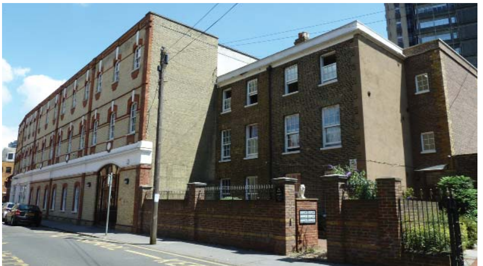
Locally listed buildings - numbers 3 (former Pickfords warehouse) and 4-5 Old Palace Road (see p.29)
