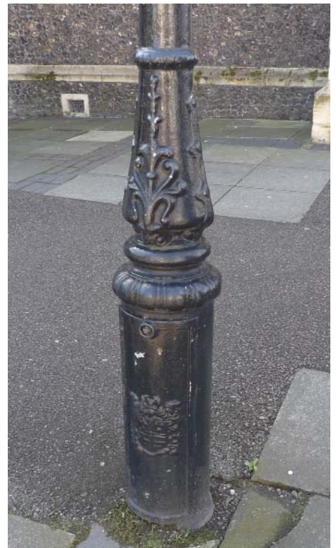
Historic street furniture in the Croydon Minster Conservation Area: detail of historic lamp column (see also p.24)
