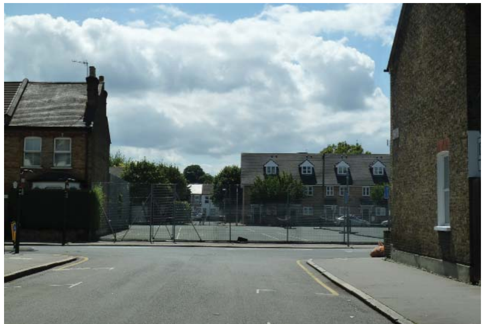
Gap site on Howley Road, as a result of World War II bombing, viewed from Old Palace Road. This site could be improved through new buildings or the frontage improved by better screening or planting.
