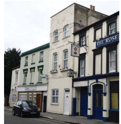
Locally listed Victorian buildings on Church Road (numbers 126-132) to the left of the Grade II listed former Rose & Crown public house
