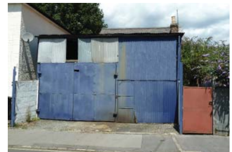
2A Howley Road, which detracts from the character of the conservation area
