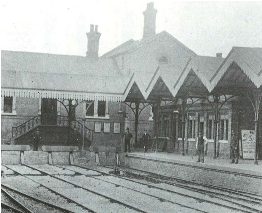
Central Croydon Station once stood on the site of the sunken area of The Queen's Gardens.
