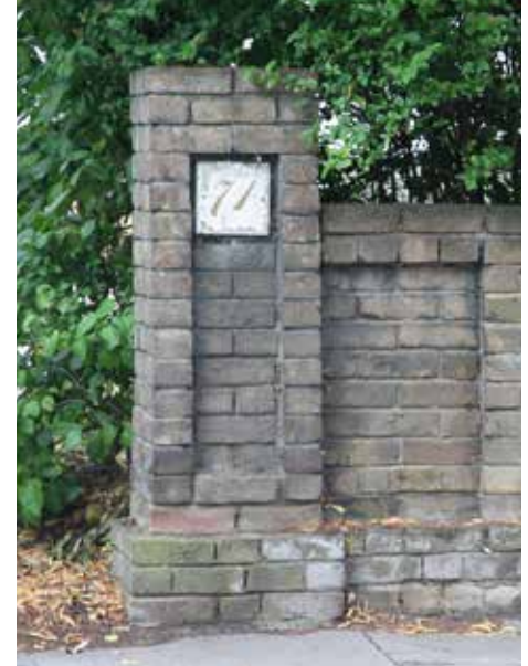
Example of brick wall boundary treatment
