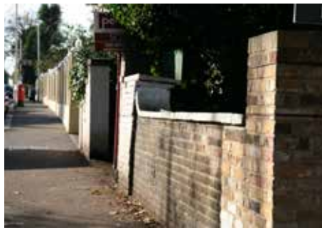
Mid level brick boundary treatment on Church Road
