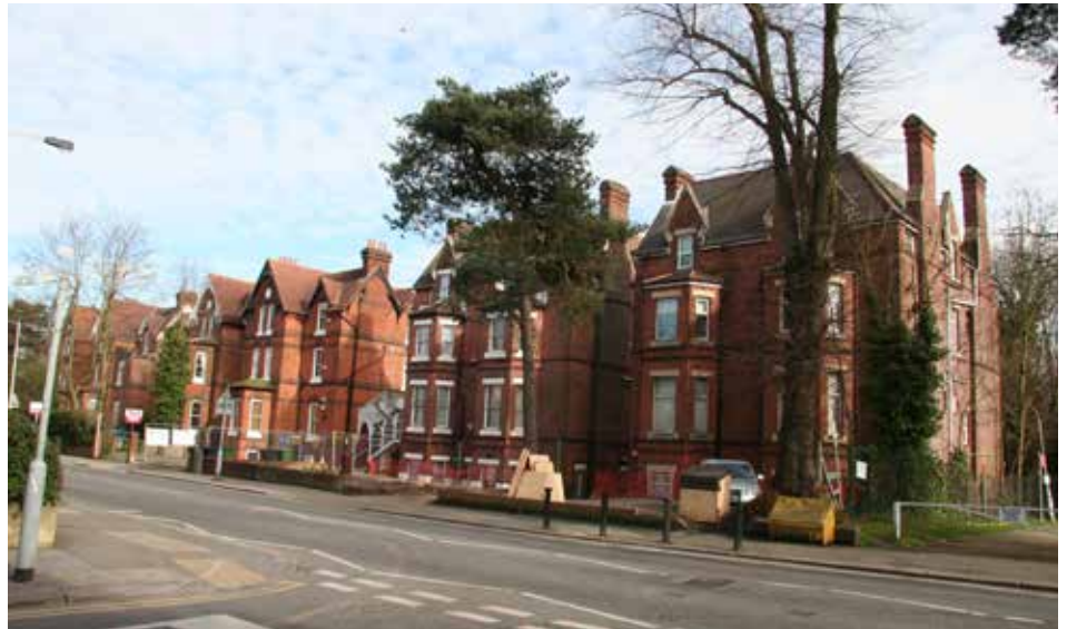
Numbers 273-281 Church Road, red brick Gothic-style villas
