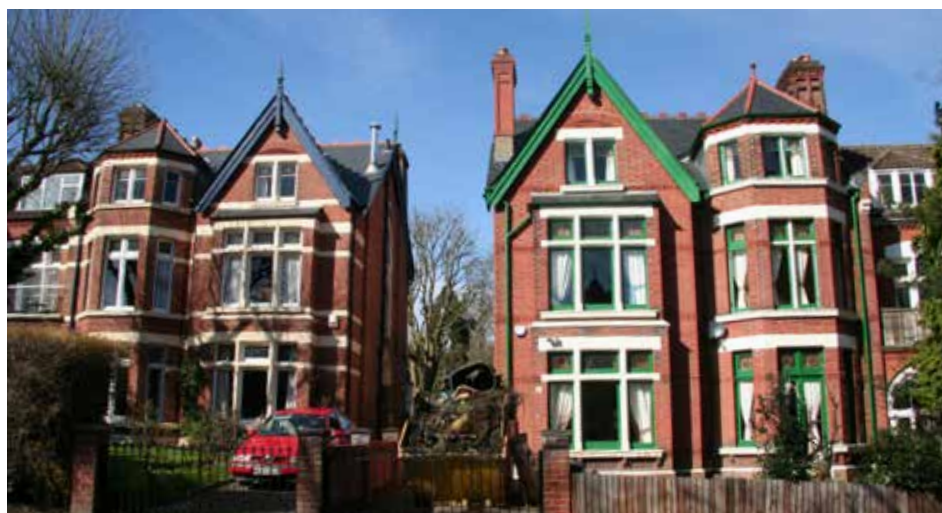
Red brick villas on Auckland Road, numbers 157-159, with parts of numbers 155 and 161 visible either side
