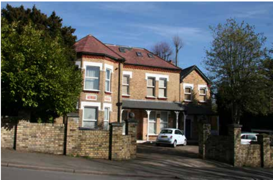
An example of a two-storey side extension to the right hand side of a building on Sylvan Hill. This extension would have been less visually intrusive if it had been set back from the front building line and had been of a smaller scale to preserve spacing between buildings
