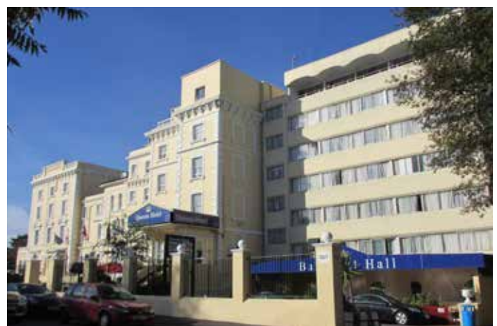
Large massing of the Queens Hotel with has a detrimental impact on the conservation area
