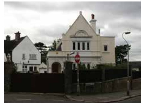
217 South Norwood Hill, turning the corner with Grange Hill
