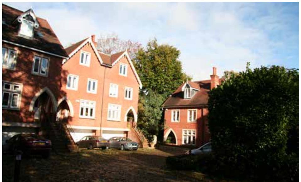
Modern cul-de-sac development at Limekiln Place on the former garden of the historic building at 153 Auckland Road, well spaced, integrated with landscaping and set around a gravel surfaced drive that contributes to the organic character of the development
