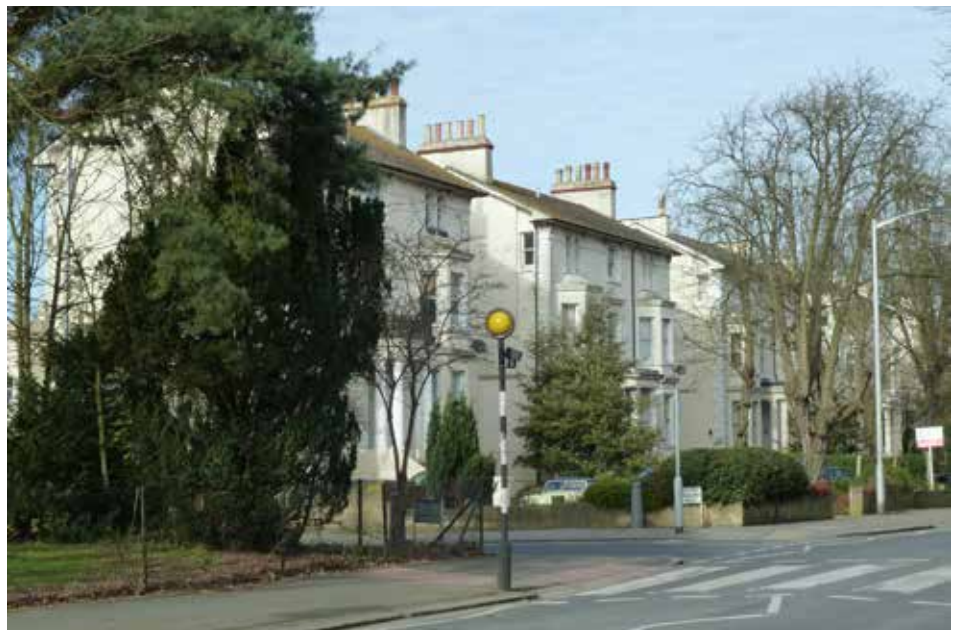
Numbers 152-158 Church Road, Italianate stucco-faced villas
