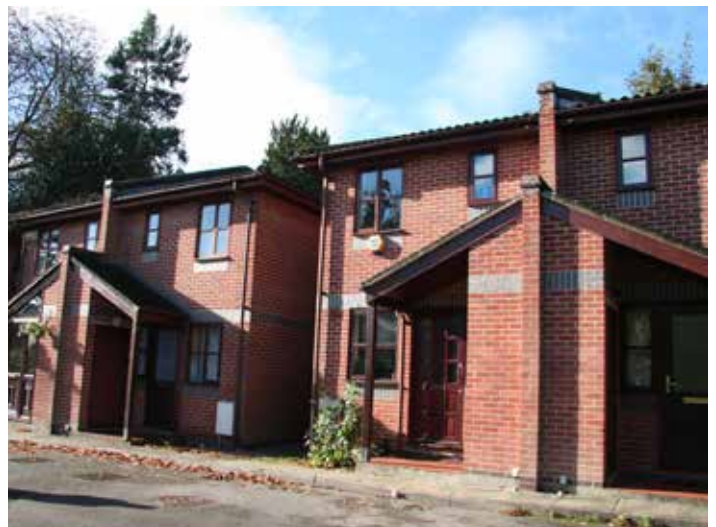
1980s development on Copper Close, a densely laid out development with poor pedestrian access and a lack of soft landscaping and trees
