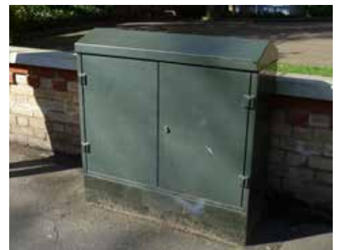
Well sited telecommunication cabinet to the rear of the footway
