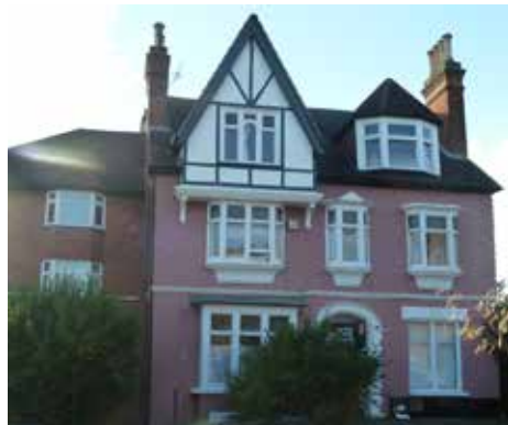
67 Harold Road with oversized side extension
