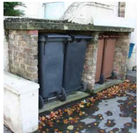
An example of good screened bin storage away from the street
