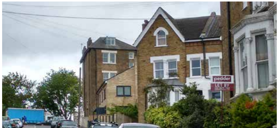
Front elevation of 1a Rockmount Road
