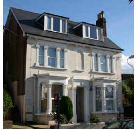
Installing dormers facing the streetscape is to be discouraged
