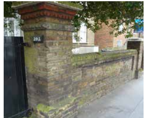
A good example of a well defined front garden boundary wall
