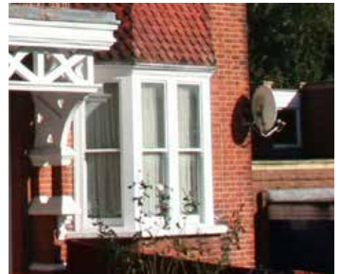
Poorly placed satellite on the right hand side of the front elevation
