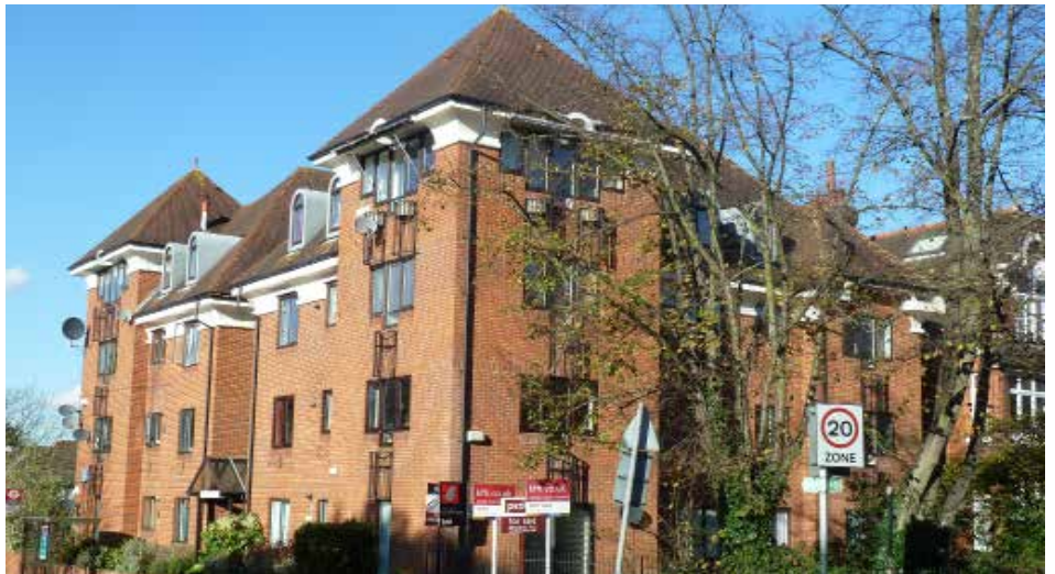
83 Chevening Road is a building which detracts from the conservation area due to its imposing scale and bulk
