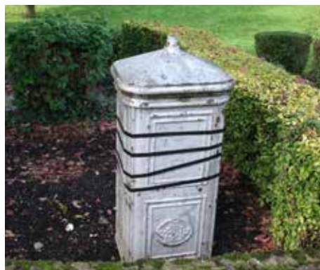
Street furniture in the recreation ground in need of maintenance
