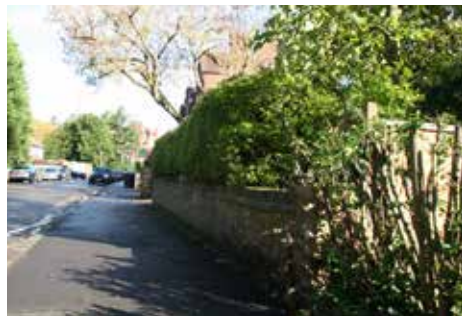
Typical soft boundary wall in the Harold Road Conservation Area
