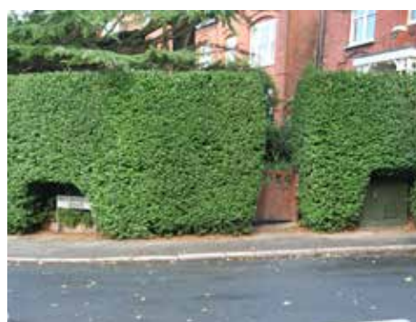
Clever pruning of hedging to accommodate telecomms cabinet in the conservation area
