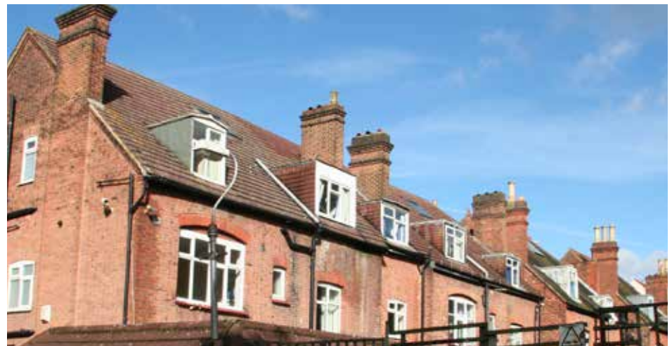
Addition of rear dormer windows breaking the rhythm of the original roof line
