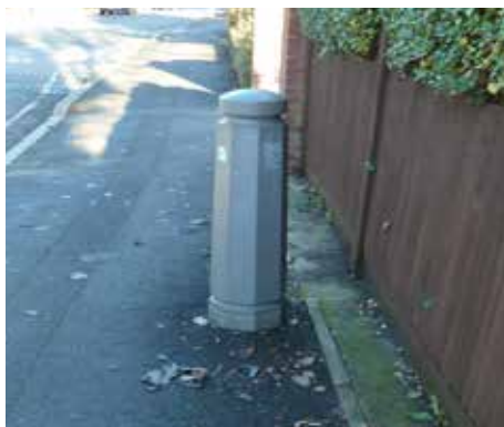
Unnecessary bollard in the Harold Road Conservation Area creating street clutter
