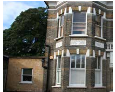
Unsympathetically designed side extension, which also blocks views
