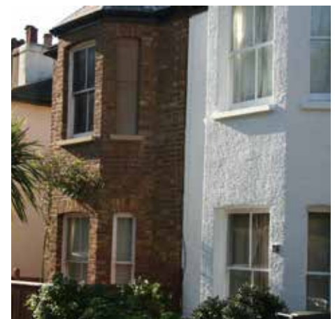
Original timber sash windows
