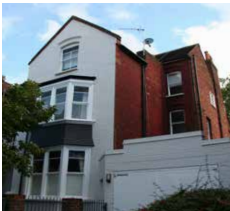
Inappropriate garage extension and painting of exposed brickwork to the front elevation
